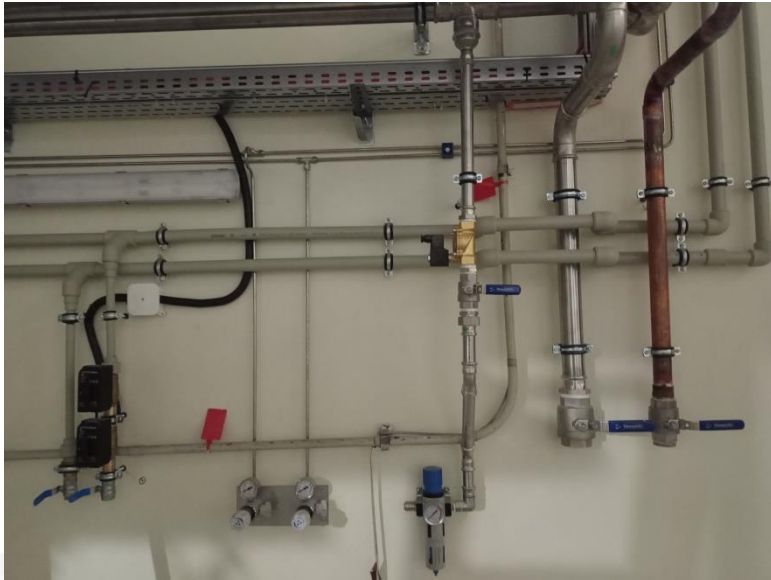
Pressurized air, He recovery, cooling water, N2 and He installations
