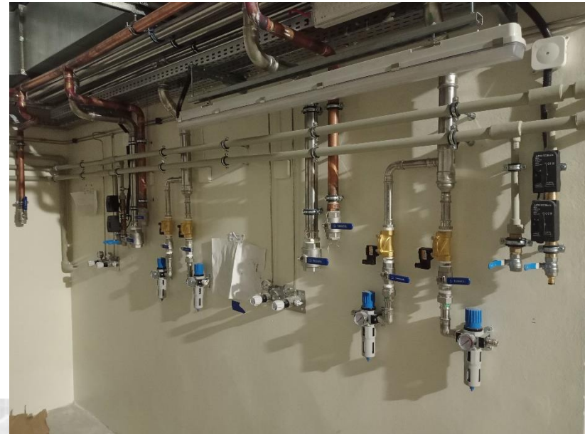
Pressurized air, He recovery, cooling water, N2 and He installations
